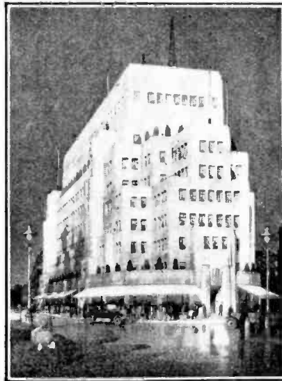
"BROADCASTING HOUSE." The approved design for the B.B.C.'s new building at Portland Place, London, W. The studios will be situated in the central block, the surrounding offices giving protection from street noises.
